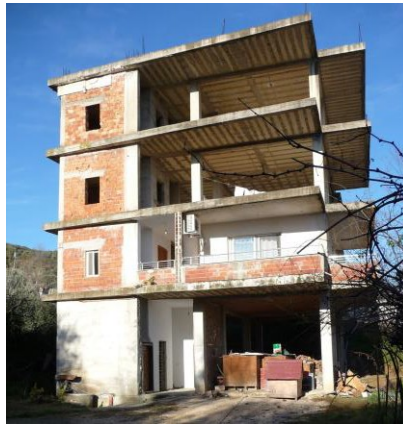
Figure 4: A reinforced concrete frame is completed and then walls are infilled
