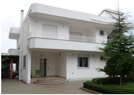
Figure 9: An undamaged house adjacent to a badly damaged building
