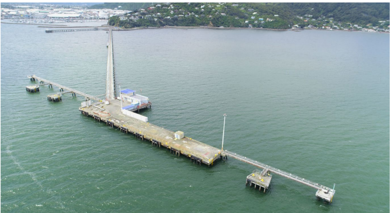
Figure 1: General aerial view of Seaview Wharf looking north-east
