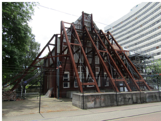
b) Old Municipal Chambers
