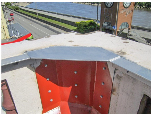
Figure 6 (left): Steel plate corner bracket and horizontal angle girts.
