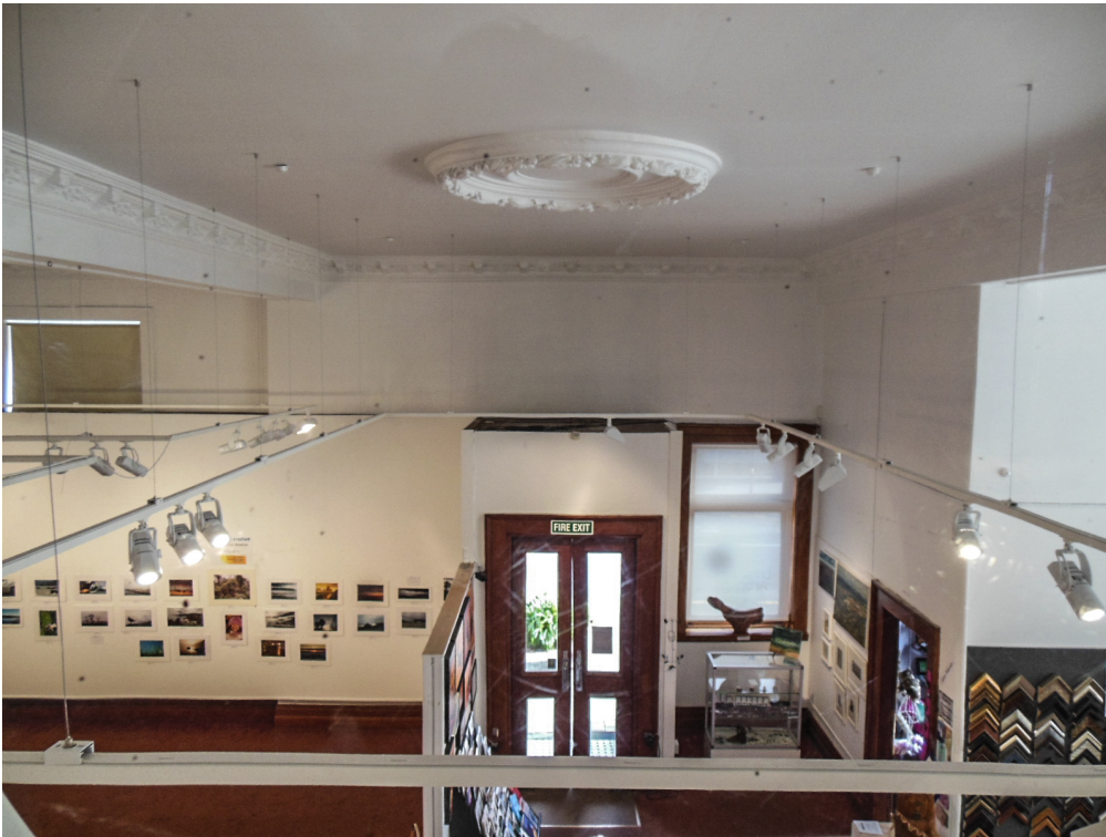
Figure 11: “Before” photo of original building prior to strengthening works being carried out.
