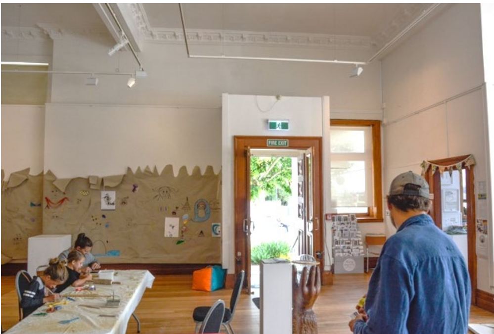
Figure 12: “After” photo of seismically strengthened building from same view.
