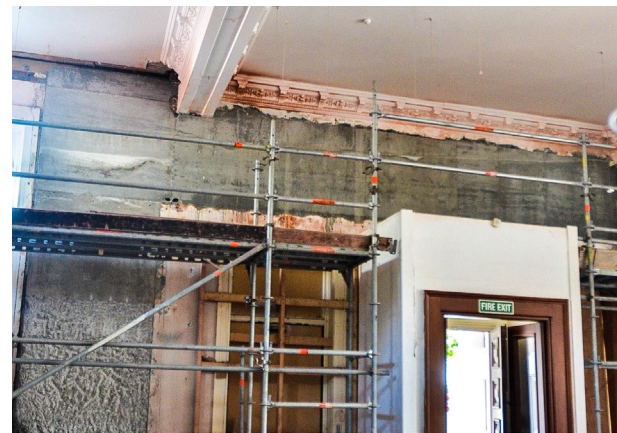
Figure 9 (left): Unreinforced masonry above the main entrance is potentially unstable in out-of-plane loading.
