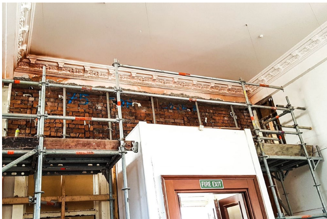
Figure 9 (left): Unreinforced masonry above the main entrance is potentially unstable in out-of-plane loading.
