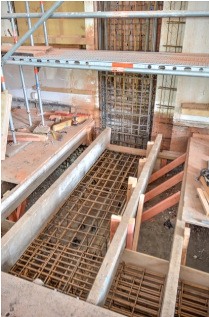
Figure 8: Sufficient monitoring took place to ensure that critical details such as beam column joints were correctly reinforced.
