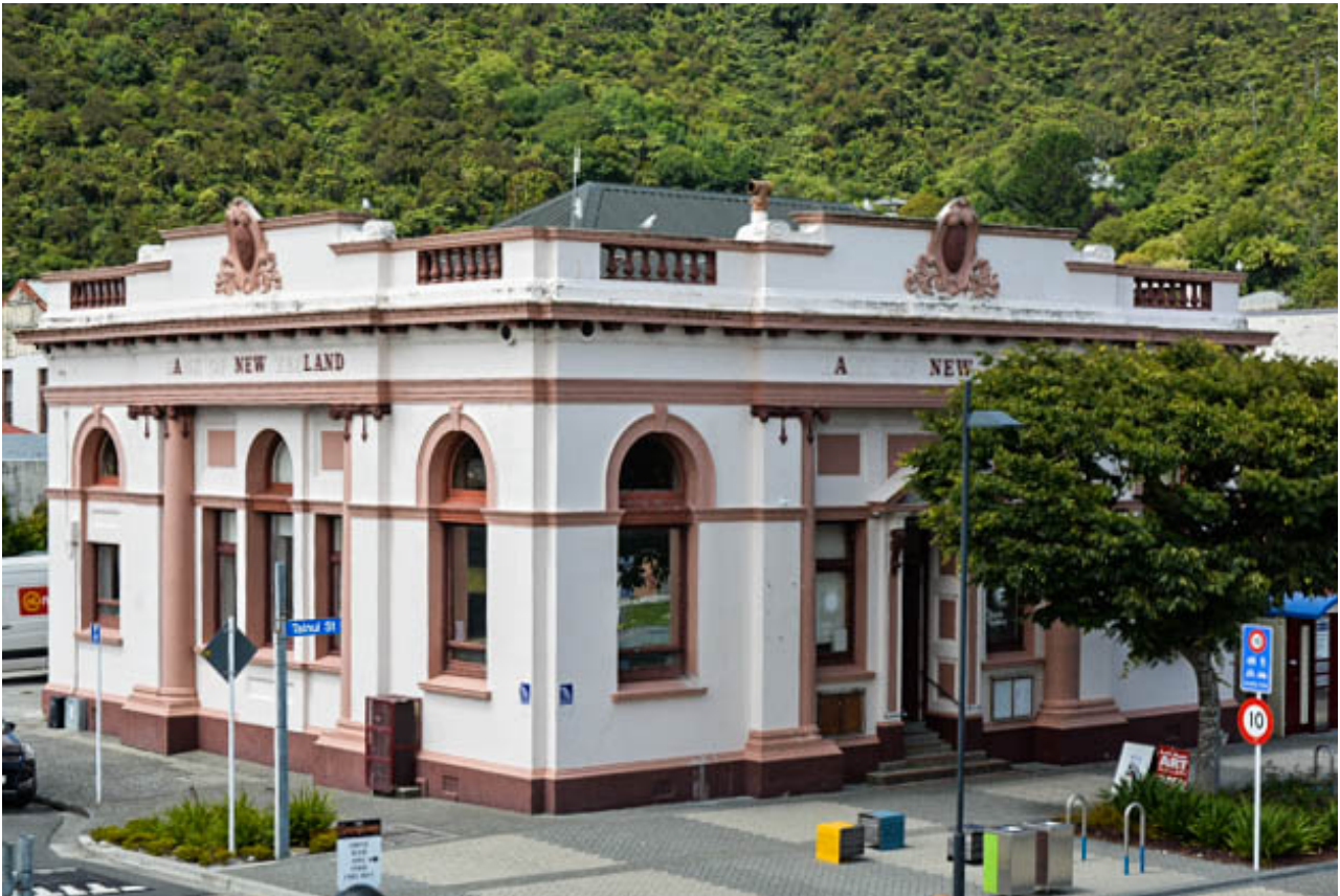
Figure 1: Left Bank Art Gallery after seismic strengthening view from the new viewing platform, 2020.
