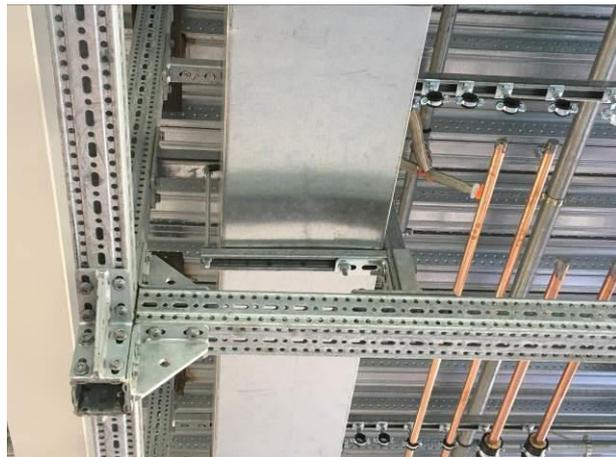
*Photographs 1 and 2- Cradle frames with installation of services occurring*
