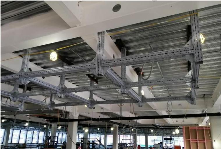
Photograph 5- Cradle frames installed prior to services installation.
