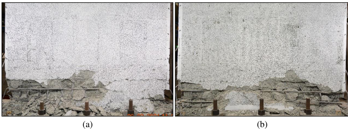
Figure 2: Damage in walls after the test, (a) W1C, and (b) W2D.
