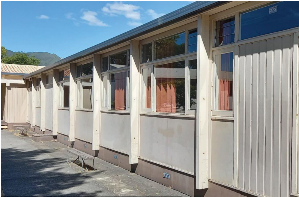
Figure 1– CEBUS block exterior (note exposed portal columns)
