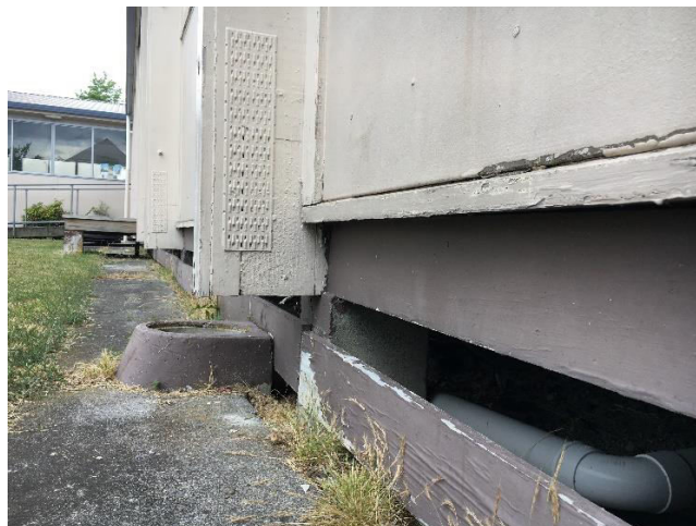
Figure 3 – Exposed portal base gangnail connections
