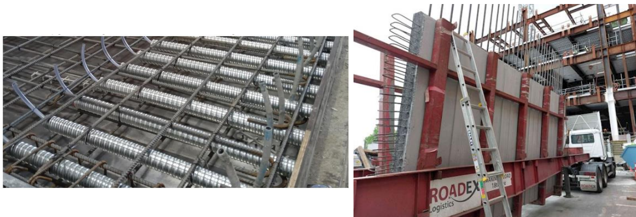
Figure 6: Panel mould prior to casting and arriving on site
