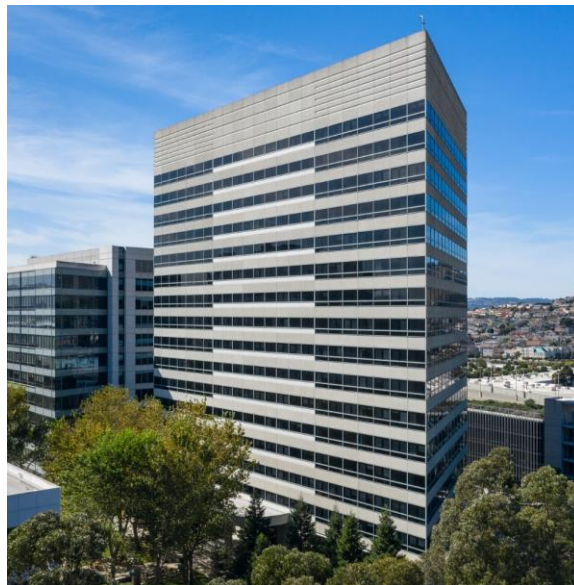
Figure 1: Pre-retrofit building at 651 Gateway Boulevard in South San Francisco, California.
