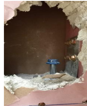
(b) exposed view of Handibrac hold-down device
