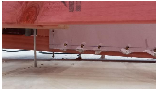
(b) Handibrac pulled out of the floor
