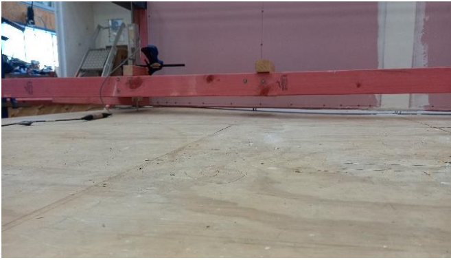
(a) Out-of-plane bowing of the floor
