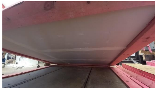
(c). Final appearance of the ceiling
