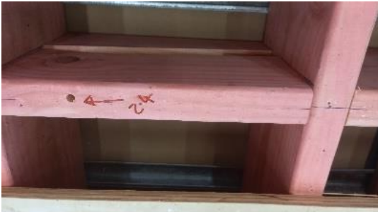
(a) Splitting of the blocking framing
