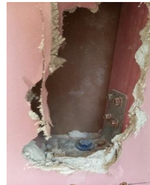
(b) exposed view of Handibrac hold-down device
