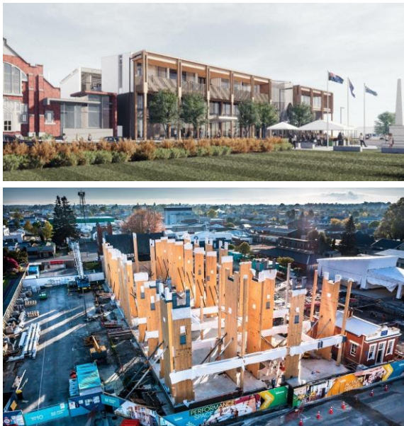
Ashburton Civic Centre – Ashburton (2020-2024)
