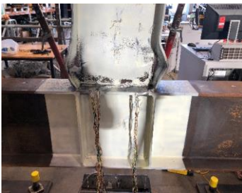
Figure 7: Large-scale tests of welded moment connections made by EFPBWs under seismic loading.
